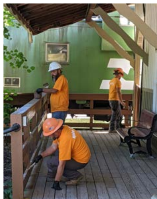
Deck work behind Barrett Station Depot
