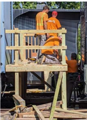
Spire workers create new ramp and platform for Train of Thought
