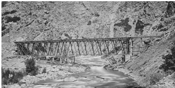
Rising water took out some of the supports for Devil's Gate Bridge over the Weber River, making it unsafe for the original Union Pacific locomotive to cross, so No. 119 got the call to go to Promontory Summit.
